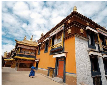
Figure 1 typical Lhasa building (Source from: http://yeschinatour.com/ )
